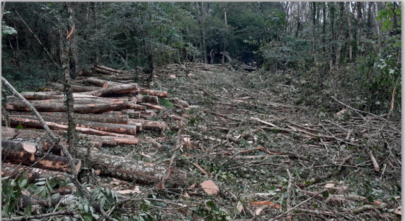
Ash clearance ready for replanting
